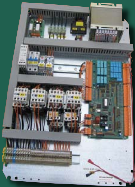
D type two speed control panel
